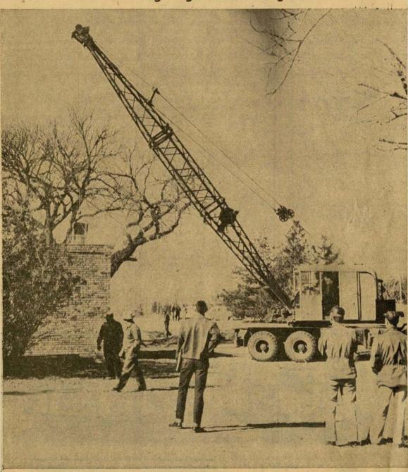
The "wrecking ball" on the end of this mobile crane made short work of the roof of this college garage this afternoon as Hunter Construction company crews began clearing land for the new Fort Hays State college Memorial Student Union. The "ball," visible just above the garage, was necessary because of the slab concrete roof. A
