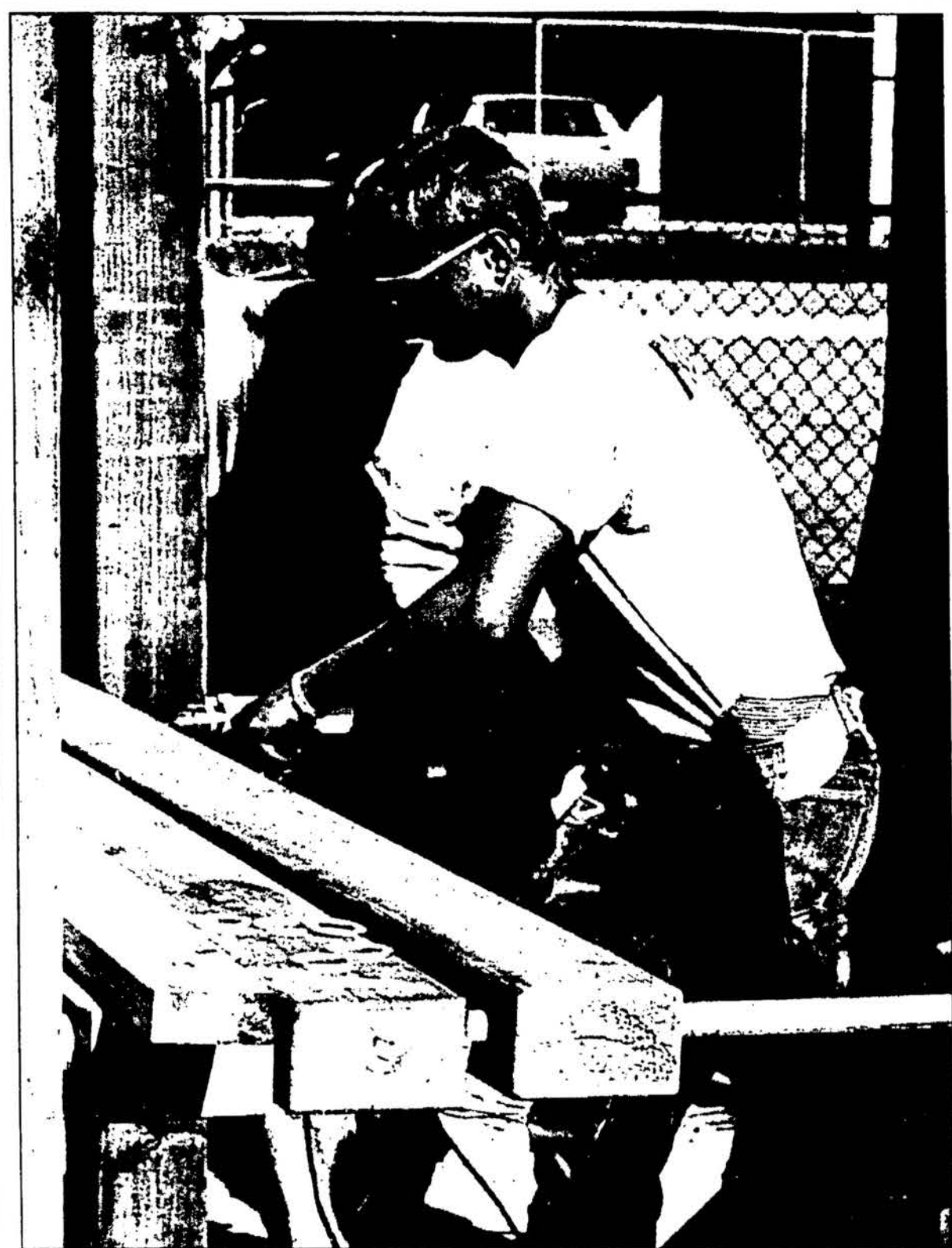
Dan Penner, Hays, and Mitch Funk, Hays, work on the new playground equipment at the Early Childhood Development Center Monday afternoon. Penner and Funk work for Paul Wertenberger Construction of Hays. The equipment was designed for both handicapped and non handicapped children since ECDC is an integrated preschool.
