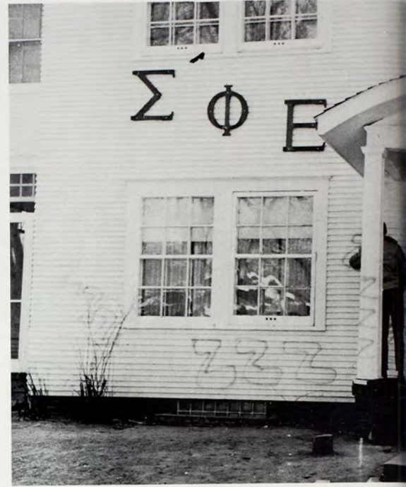
Sig Eps examine the damage to their house, which was inflicted during the night by vandals.
