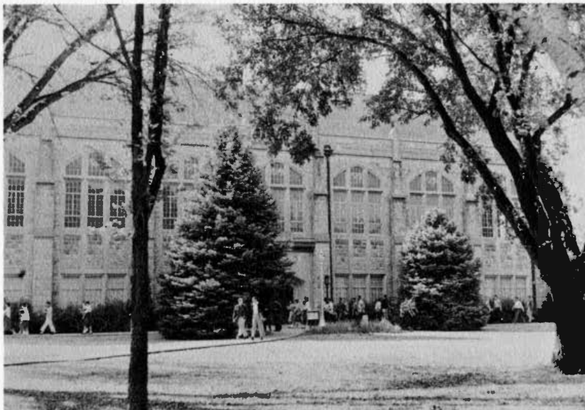
The exterior of Forsyth Library today.
