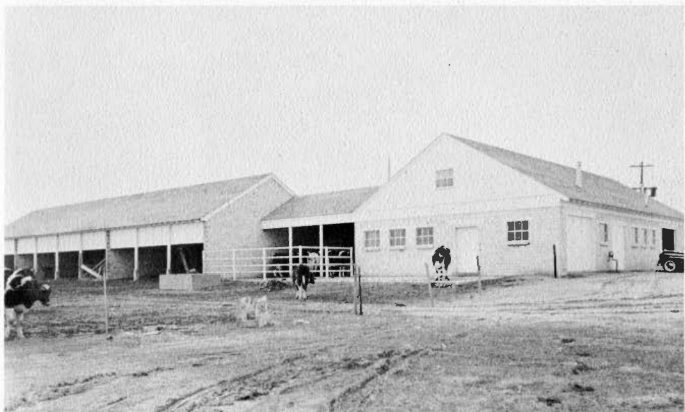
Modern buildings and equipment have replaced the old facilities on the college farm.
