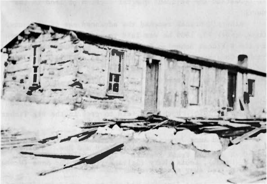
Stone and log house built by Frank Mazanek after he moved from his sod house.
